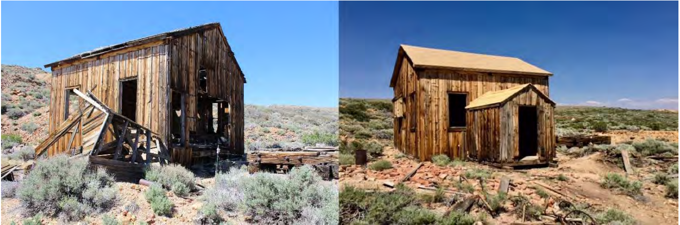
Bodie Hoist House, CA. 2018. Before (left) and after (right) Bodie Foundation and California State Parks System
